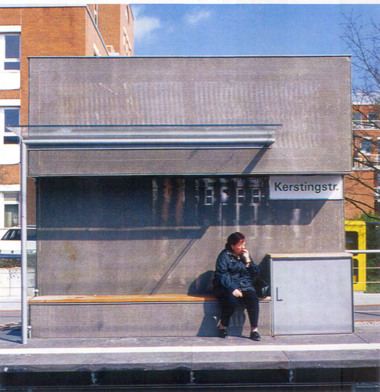
Below: Kerstingstrasse station: made with fine stainless steel mesh.
