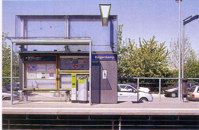
Above: The cladding reflects the texture of local buildings or landscape.
