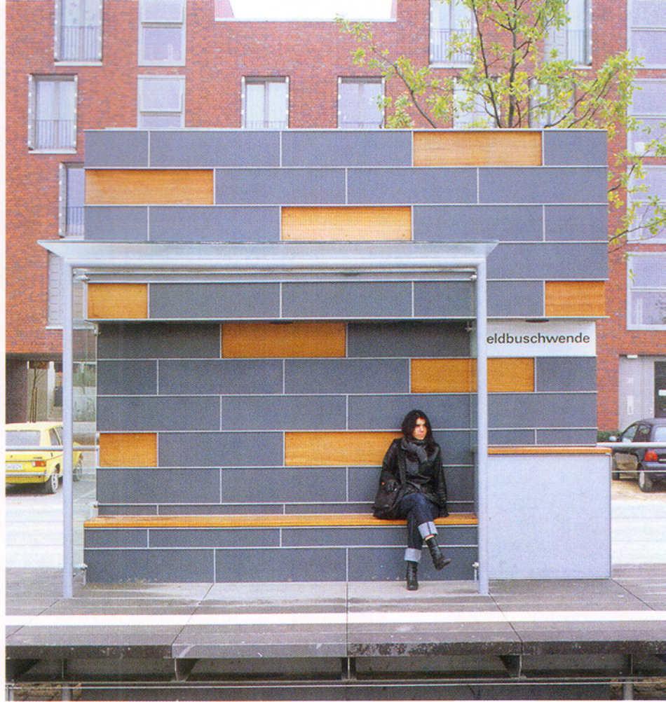
Below: Kronsberg station: made with pebble cladding.
