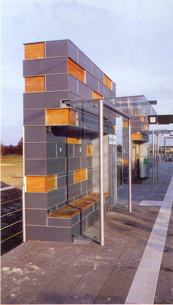
Above: Feldbuschwende station: made with a mix of metal (plates) and timber.
