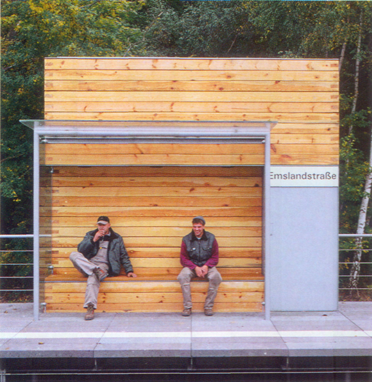
Above: Emslandstrasse station: made with timber.
